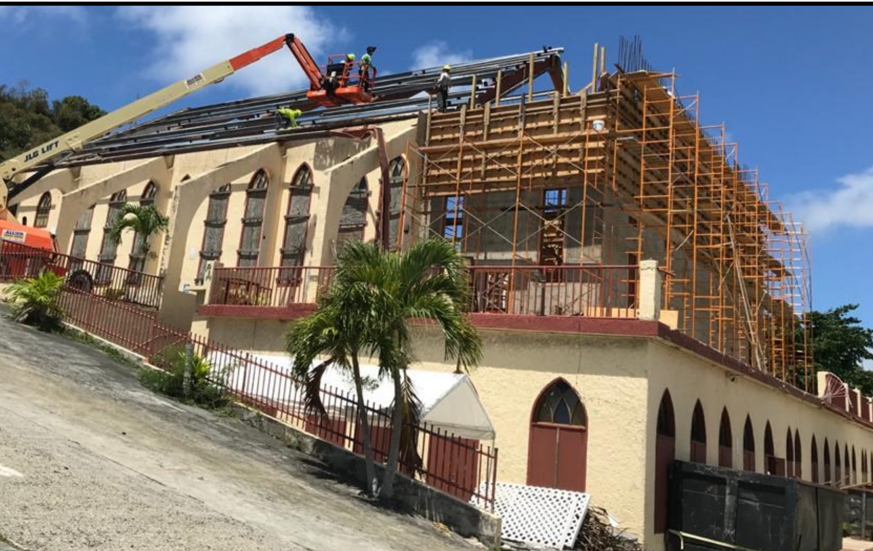
The church now under construction was destroyed by Hurricane Irma 2017
