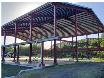
Southern Academy - Multipurpose Hall Project Under Construction
